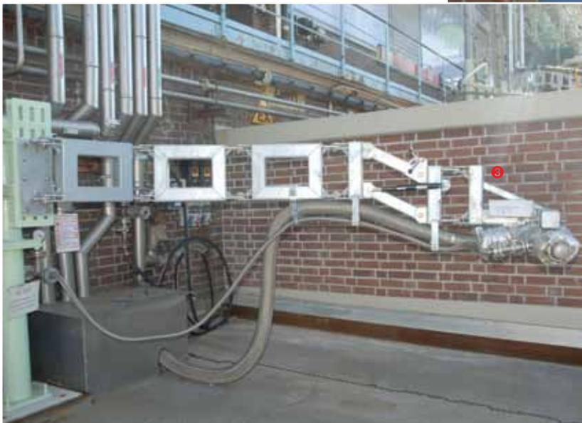
**Hose loading arm (4.37 m) for a heavyweight class hose line with a weight of more than 100 kg.**
